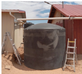
Installing rainwater roof catchment tanks and water sampling
